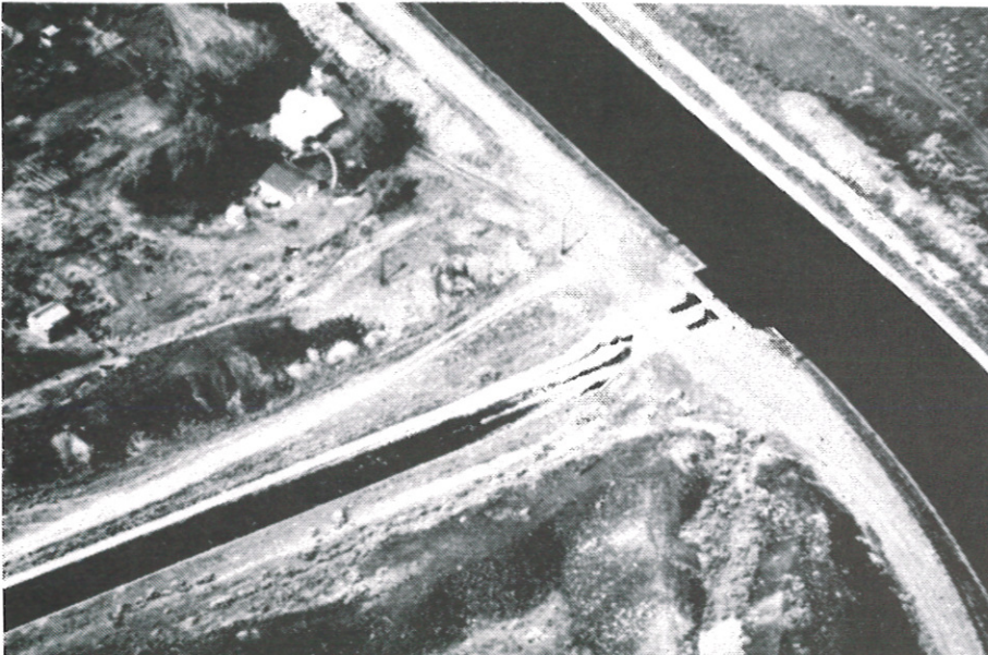
EAST LOW CANAL outlet structure is dilution water release point into Rocky Coulee Wasteway
