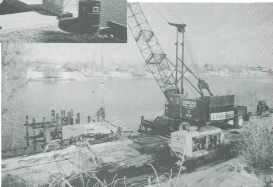
PARKER HORN PUMP STATION under construction
